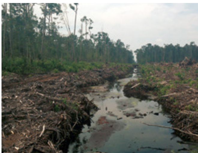
21 March 2016, PT Persada Kencana Prima: 3°42'05.85"N 117°04'24.47"E: drainage canal, recent deforestation and young oil palm saplings. ©Aidenvironment
