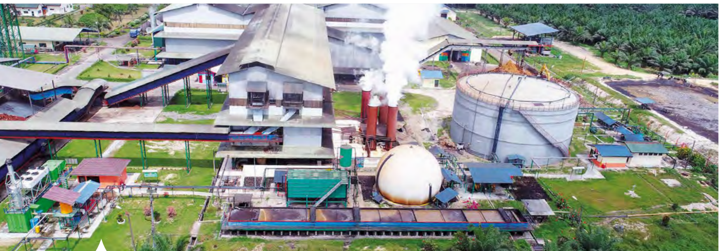
Biogas power plant at an Indonesian palm oil mill
