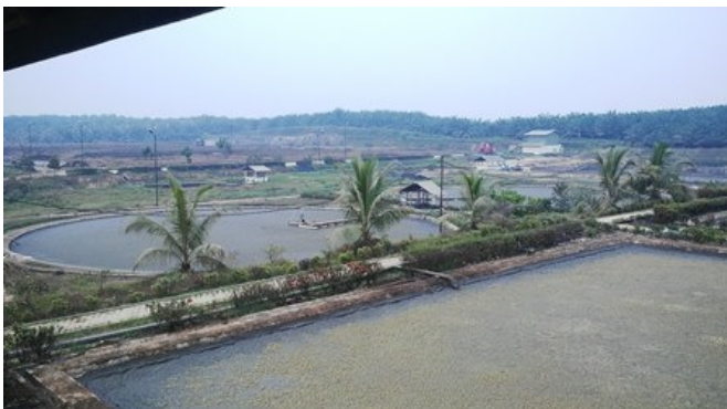
Palm oil mill effluent (POME) ponds at the PT Nirmala Agro Lestari mill in Lamandau District. DOE's SERIG project developed technical and economic analysis for generating renewable electricity from the biogas emitted from the effluent ponds at this and another nearby mill. This would provide power for the mills and nearby communities.
