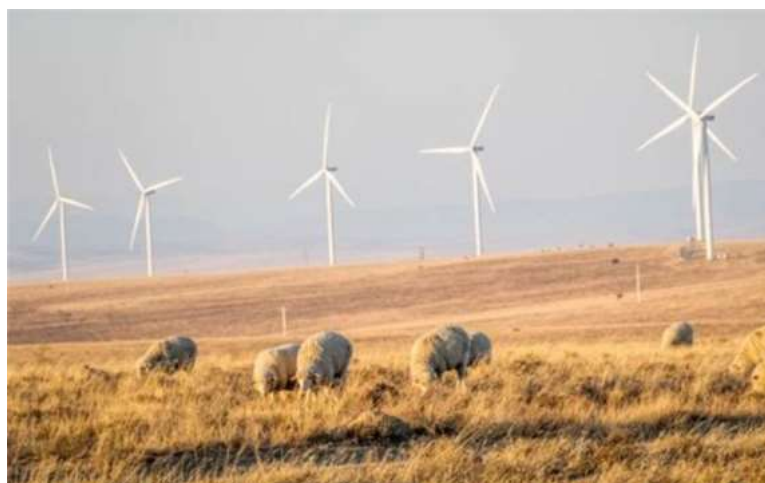
Golden Valley Wind Energy Facility. Source BioTherm Energy
