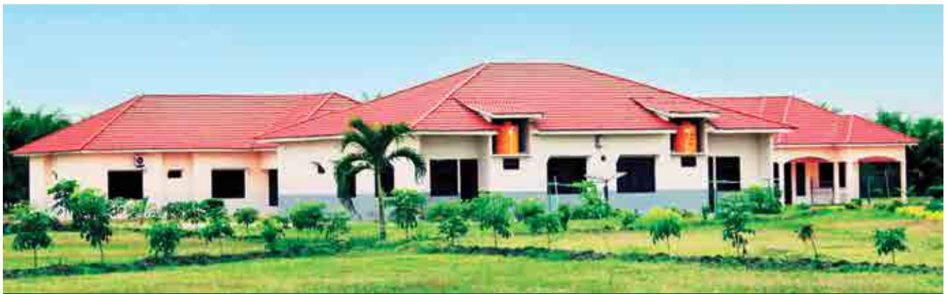
Employees’ quarters at one of KLK plantations in Indonesia
