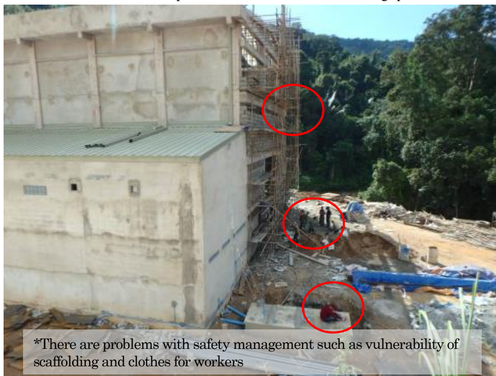
Photo 11.3 Status of powerhouse construction site at Nam Ngiep 2C
