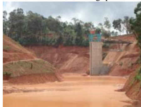
Photo 4.2 Dam Site for Nam Ngiep 2C
